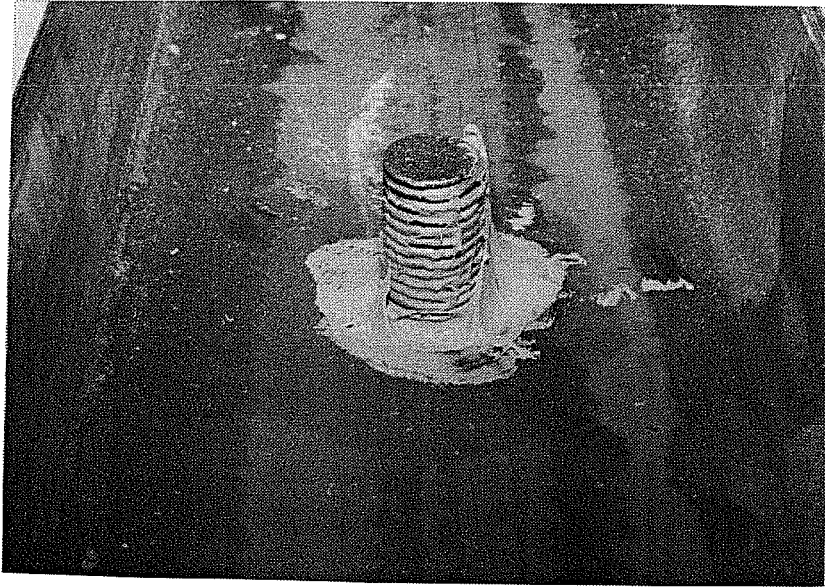
Figure 3.21 Channel in position with extruded adhesive
