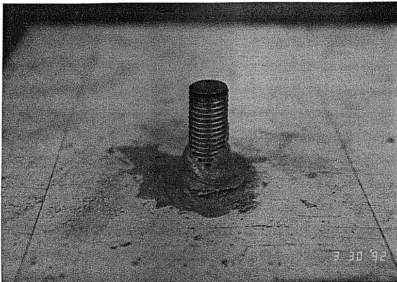
Figure 3.20 Epoxy applied to base of anchor bolt
