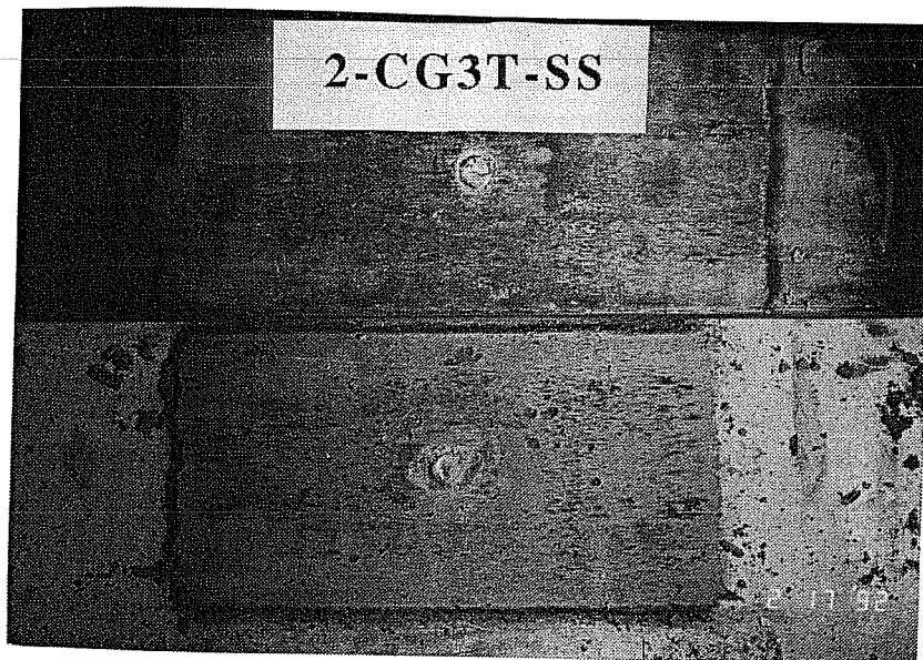
Figure 4.67 Grout interface after failure - Test 2-CG3T-SS
